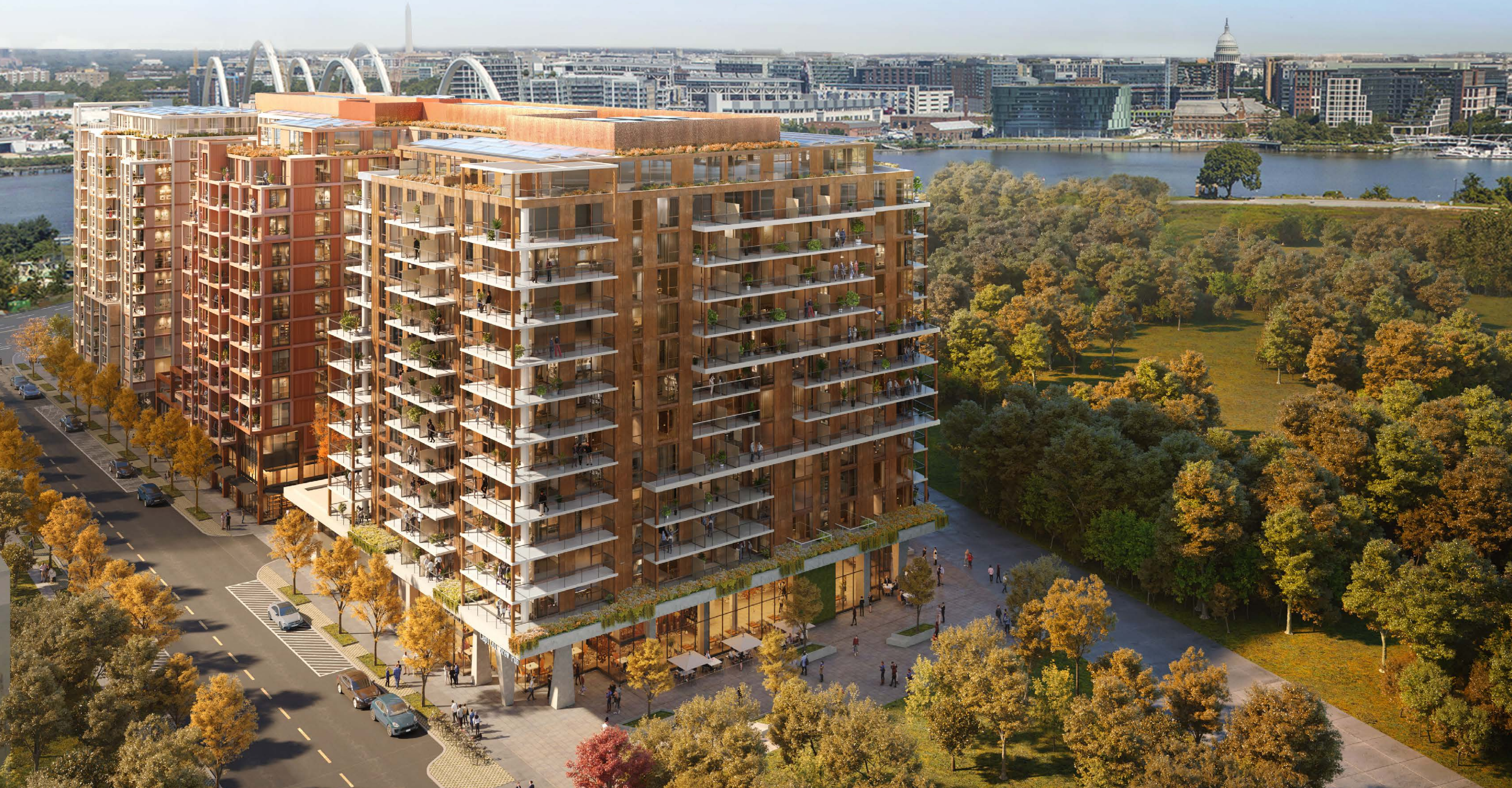
The Douglass: Aerial from South West
